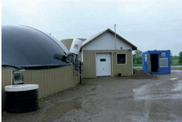
Fig. 1: Picture of Initial Fepro Farms Digester
