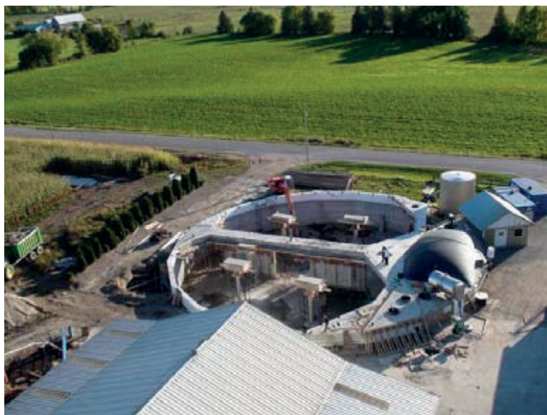
Fig. 4: Fepro Farms Larger Digester under Construction
